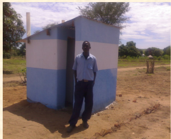
One of the Ventilated Pit latrine Built with Support from RFDP at Kazembe Basic School – In Lundazi District.
